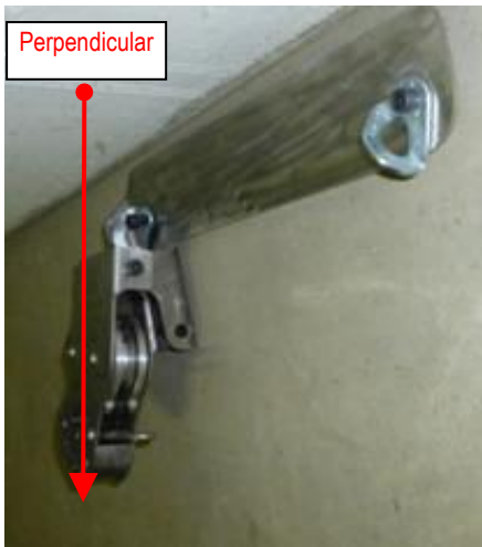
Example photo: correct wall installation with mounting bracket with horizontal fixtures
